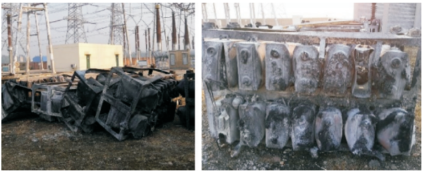
图2 1号并联电容器组现场检查 Fig. 2 Field inspection of 1# shunt capacitor bank
